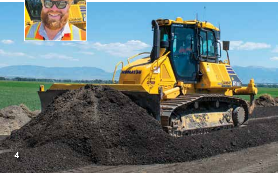
Superintendent Cody May grades a road with a Komatsu D61EXi-24 Intelligent Machine Control (IMC) dozer. "The intelligent machines increase productivity and efficiency by cutting down the time to set grade and check grade," said Cody.
