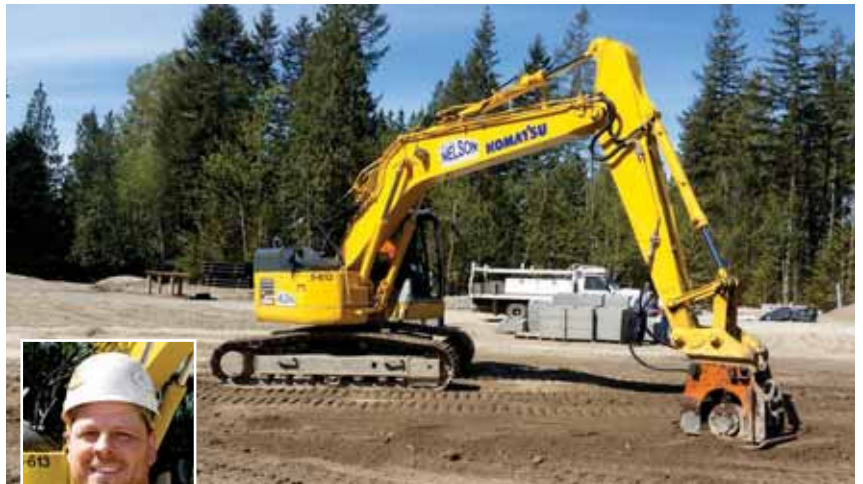
Foreman Rick McGinnis compacts soil using this Komatsu tight-tail-swing excavator. "I like our Komatsu equipment a lot," said McGinnis. "The excavators are outstanding."
