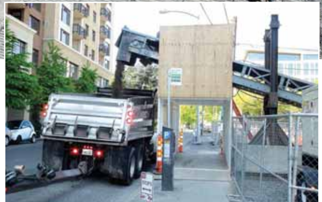
(Clockwise from bottom left) Mickelo Construction uses a Komatsu PC308 excavator to load material into a feeder that delivers it to a conveyor setup. The Spomac conveyor consists of two 36-inch belt units, one 100 feet long and the other 80 feet long. The conveyor carries material from the hole and drops it into trucks at street level. A shipping container without doors allows pedestrians to use the sidewalk throughout the excavation process.
