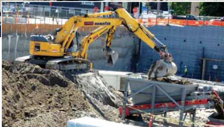
(Clockwise from bottom left) Mickelo Construction uses a Komatsu PC308 excavator to load material into a feeder that delivers it to a conveyor setup. The Spomac conveyor consists of two 36-inch belt units, one 100 feet long and the other 80 feet long. The conveyor carries material from the hole and drops it into trucks at street level. A shipping container without doors allows pedestrians to use the sidewalk throughout the excavation process.
