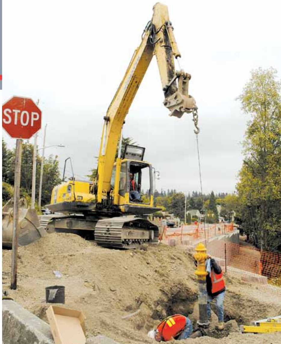
This SCI crew uses a Komatsu PC200LC-7 to help set a fire hydrant as part of a street rehab job associated with the Sound Transit light-rail project near Sea-Tac Airport.
