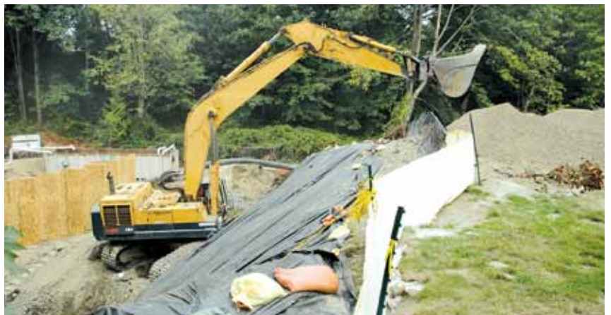
SCI rented this Komatsu PC1000 from a friendly competitor to do some deep, heavy pipe work on the light-rail job.
