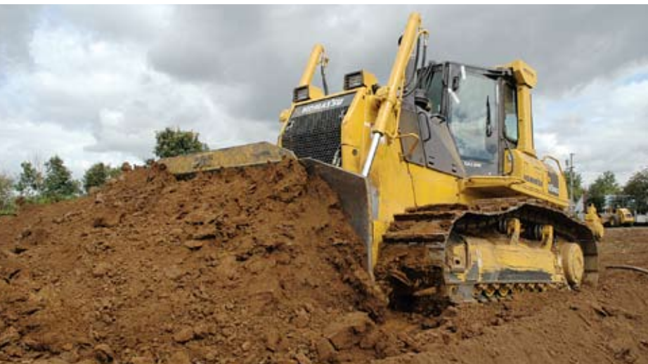
This Stacy and Witbeck operator uses a Komatsu D65WX dozer (six-way blade) to push dirt as part of the I-205 light-rail project in Portland.
